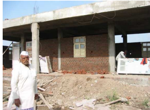
Construction of Chitgopekar School Project
