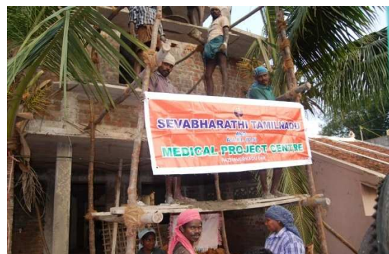
Construction Phase of Pazhaverkadu Medical Center
