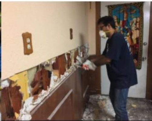
Cleaning and fixing of flooded home
